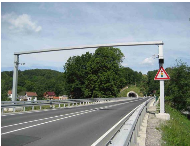
Figures 4a/b. The LS 96 One-way Light Beam Devices from Leuze electronic installed by engineering firm Keller on the columns of the sign gantries fulfill the functions of the red and white aluminum rails – here at the entrance to the Pörzberg Tunnel, the new Schaala local bypass near Rudolstadt.
