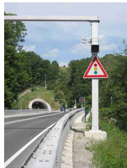
Figures 4a/b. The LS 96 One-way Light Beam Devices from Leuze electronic installed by engineering firm Keller on the columns of the sign gantries fulfill the functions of the red and white aluminum rails – here at the entrance to the Pörzberg Tunnel, the new Schaala local bypass near Rudolstadt.
