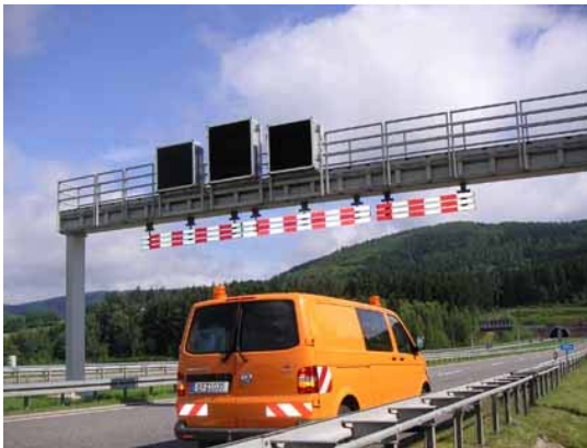
Figures 3a/b/c. Mechanical systems can be easily damaged by collisions, and several replacements a year due to damage is not uncommon. In addition, they are much more expensive than optical solutions.
